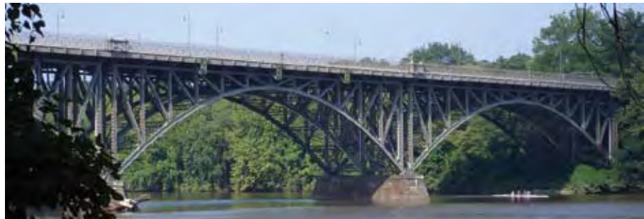
Strawberry Mansion Bridge
