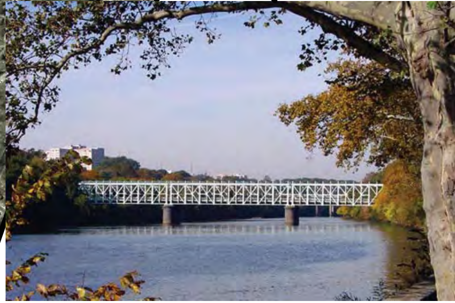
East Falls Bridge
